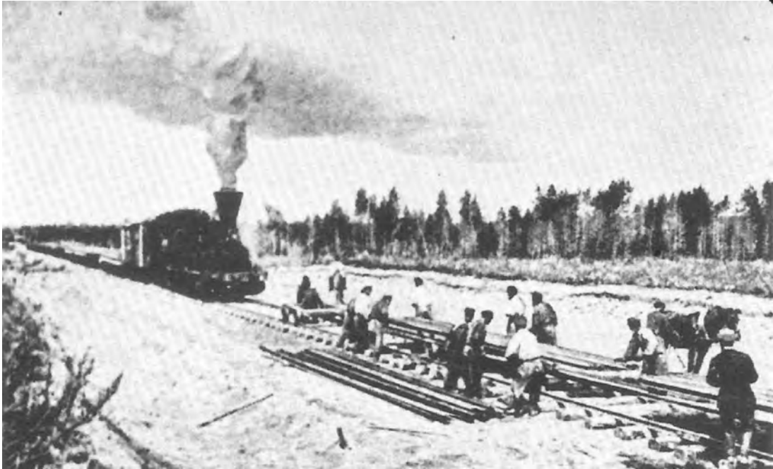
Russian workers laying the final lengths of track for the Trans-Siberian Railway.
